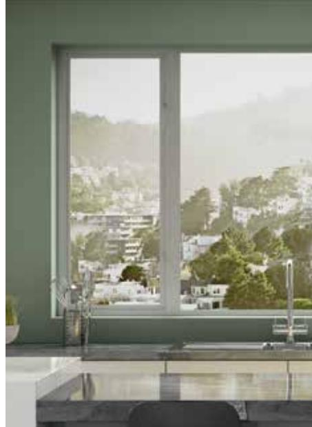
A casement window is hinged at the side and opens outward like a door. Unlike single hung or sliding windows, a casement window has no rail, providing an unobstructed view. If you're installing windows over a sink, countertop or appliance, a casement window with a crank can be the perfect solution.
