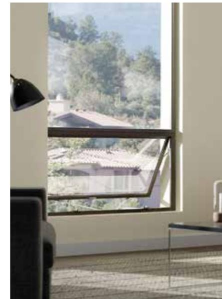
Awning windows are hinged on top and open outward, enabling ventilation without letting in rain or falling leaves. They are a great choice to pair with non-operable windows, such as above or below a picture window.
