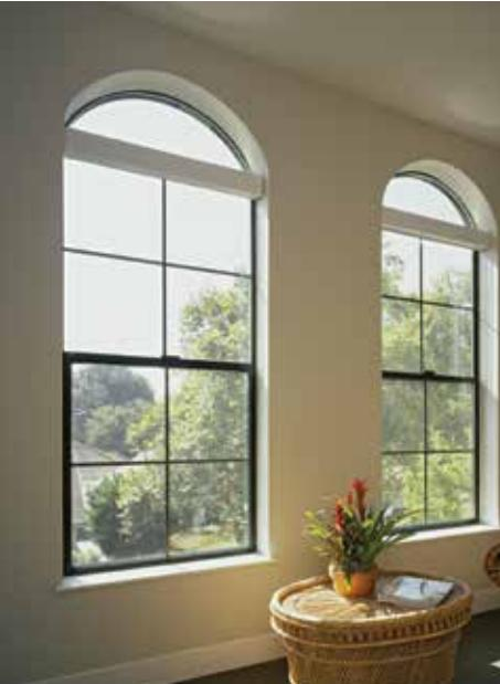
In the single hung window, the bottom sash moves up to open and allow in air flow and the top sash is fixed. Since it opens and closes without protruding, single-hung windows are an excellent choice for first-story rooms. Single hung windows work well in combinations.
